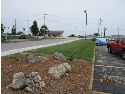
3. Backfill behind sidewalk to match grade.
