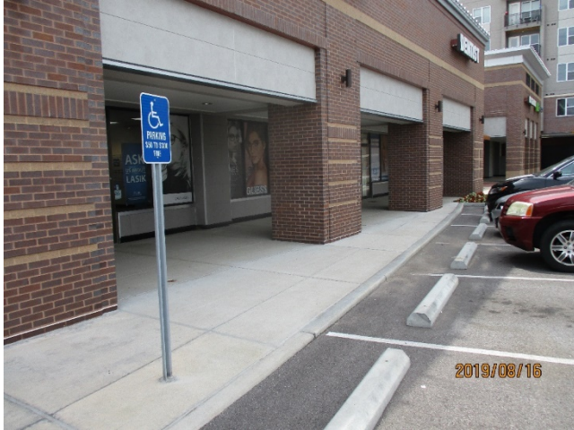
17. The plan shows 4 planters along the front of the existing commercial building. Provide planters as shown on the plan.
