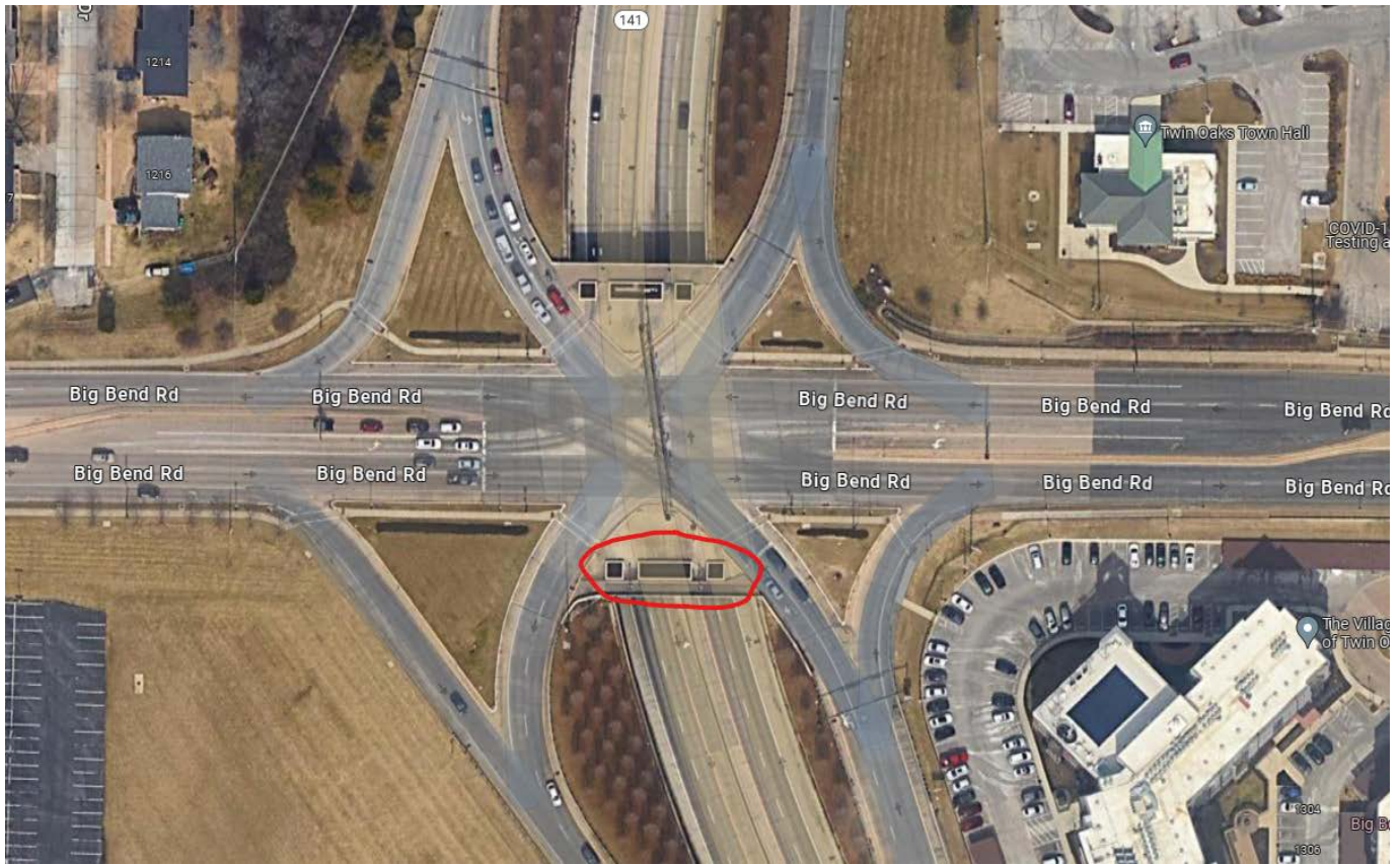
Circle indicates planter boxes to be repaired.
