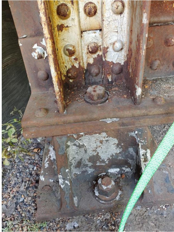
Photo 13 – Existing Steel Plate Girder (Showing Bearing)
