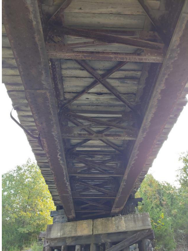
Photo 9 – Existing Steel Plate Girder (From Below)
