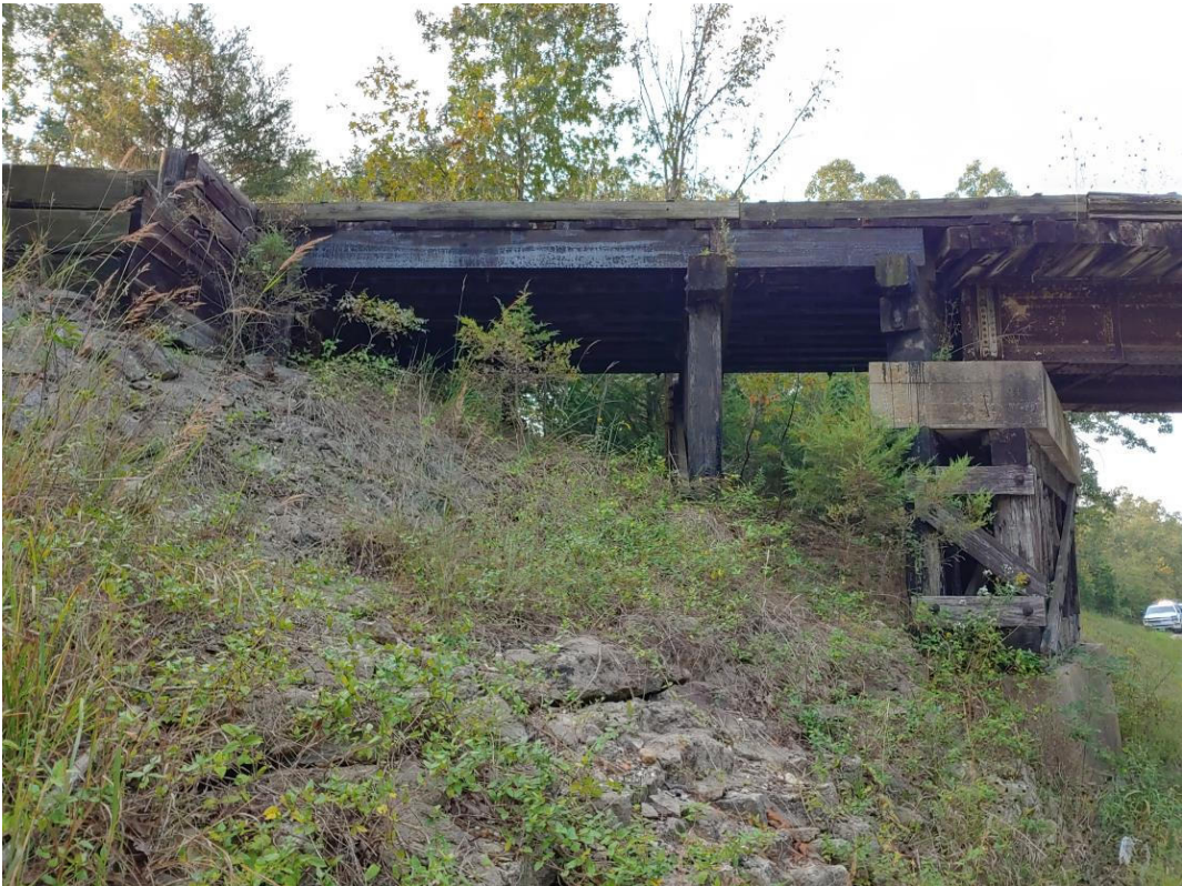
Photo 14 – Existing Timber Approach Spans
