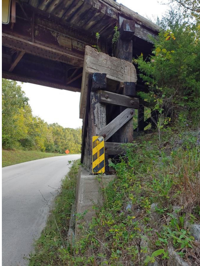
Photo 27 – Existing Interior Bent (Looking North)
