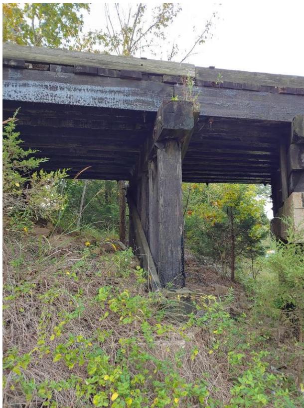
Photo 24 – Existing Timber Pier
