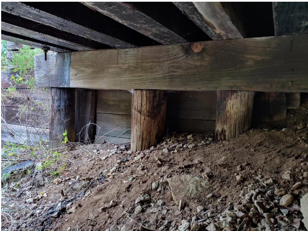
Photo 16 – Existing East Abutment Elevation (Showing Timber Retaining Wall)
