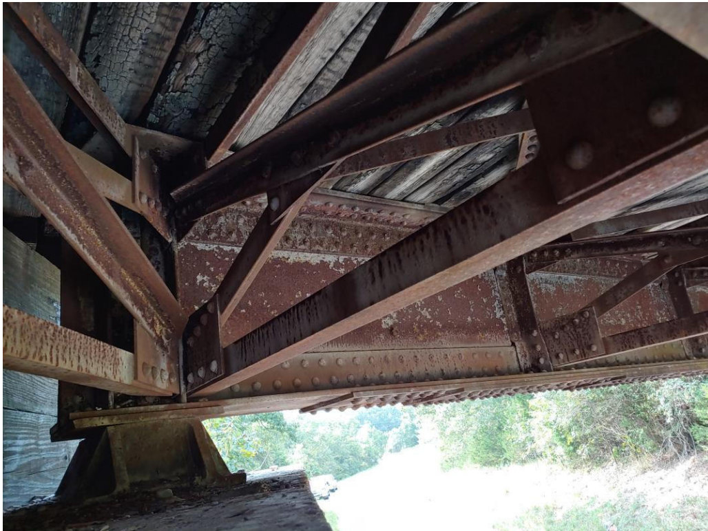
Photo 12 – Existing Steel Plate Girder (Showing Cross Frames)
