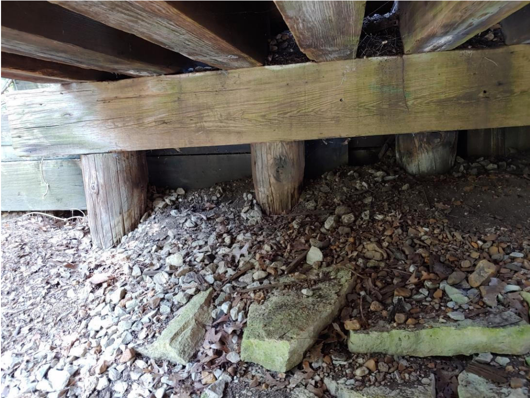
Photo 19 – Existing West Abutment Elevation
