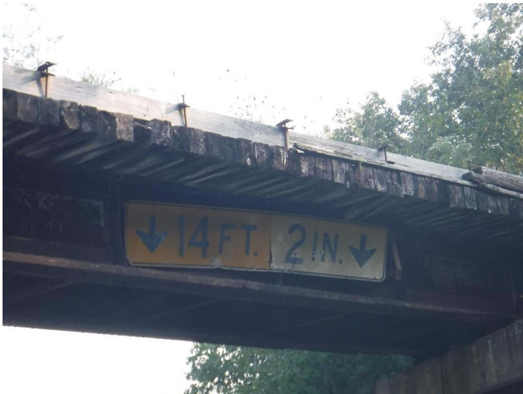
Photo 28 – Existing Roadway Clearance Sign
