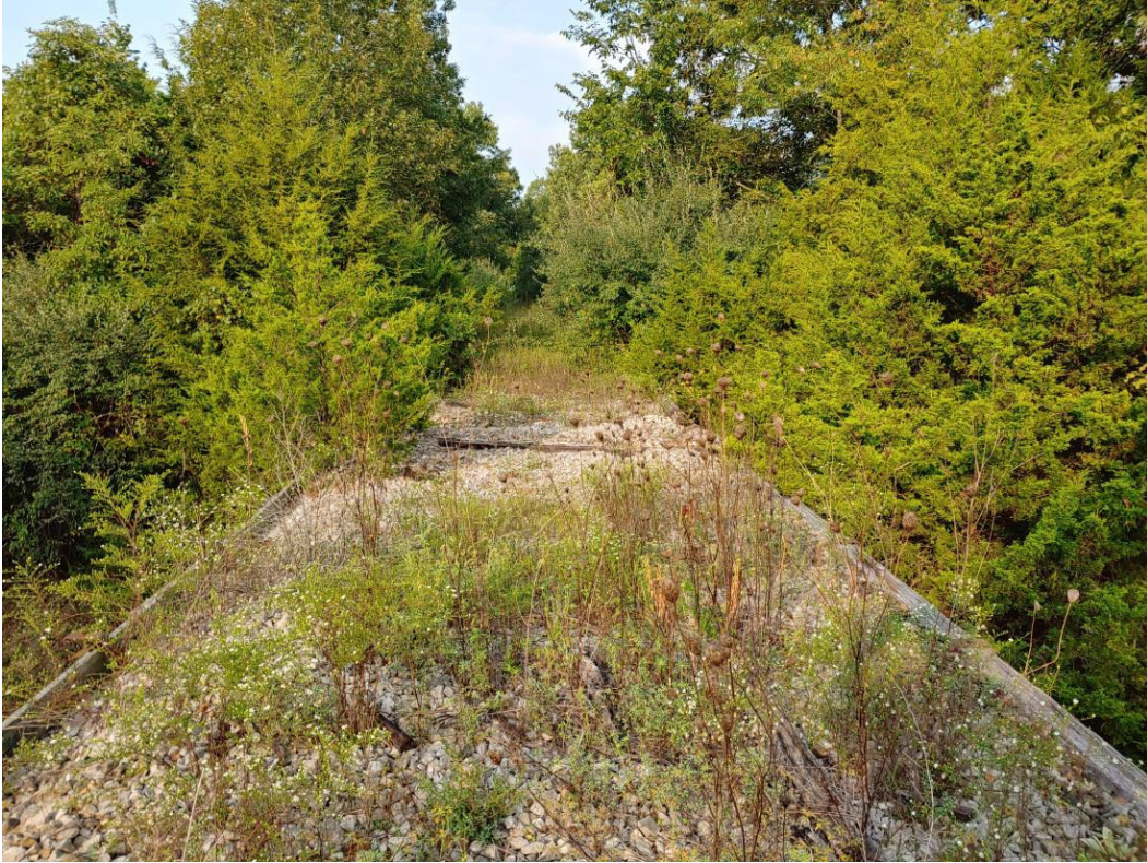
Photo 5 – Top of Bridge (Looking West)
