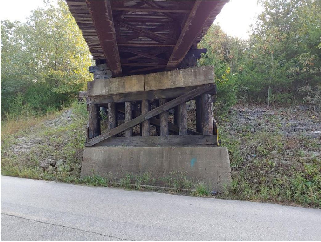
Photo 25 – Existing Interior Bent Elevation
