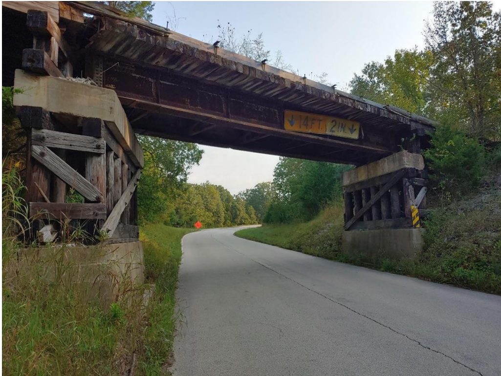
Photo 2 – Bridge Elevation (Looking North)
