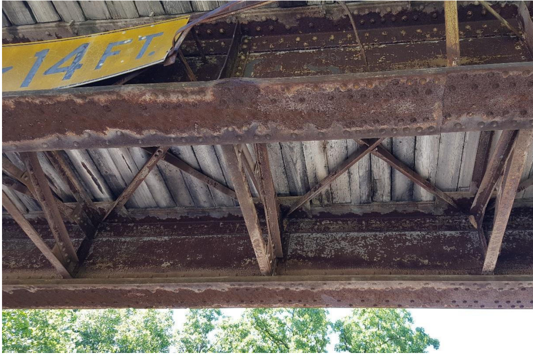
Photo 11 – Existing Steel Plate Girder
