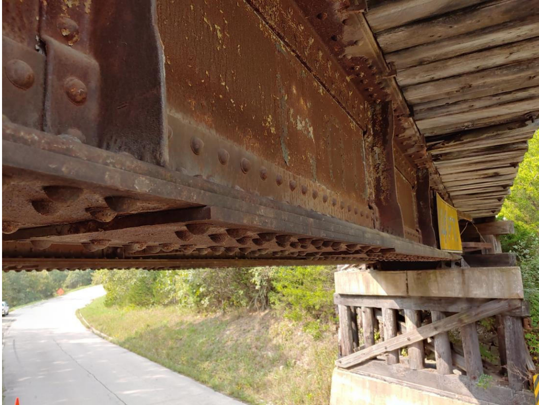
Photo 10 – Existing Steel Plate Girder
