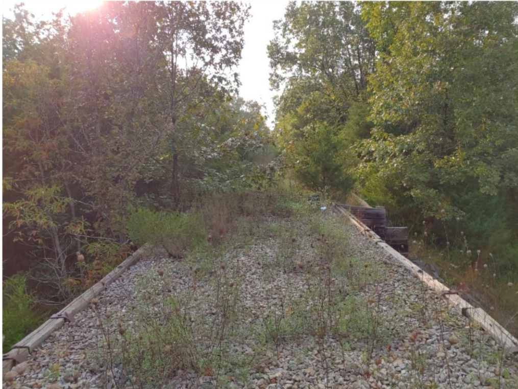
Photo 4 – Top of Bridge (Looking East)
