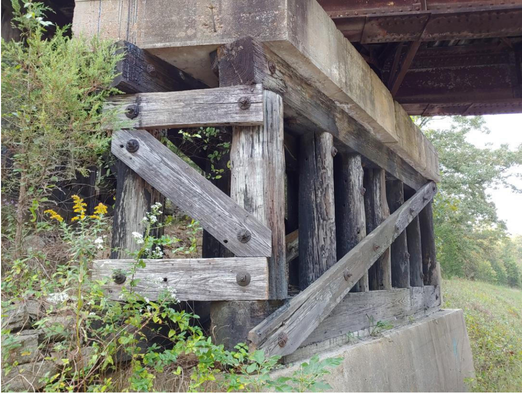
Photo 26 – Existing Interior Bent (Looking South)
