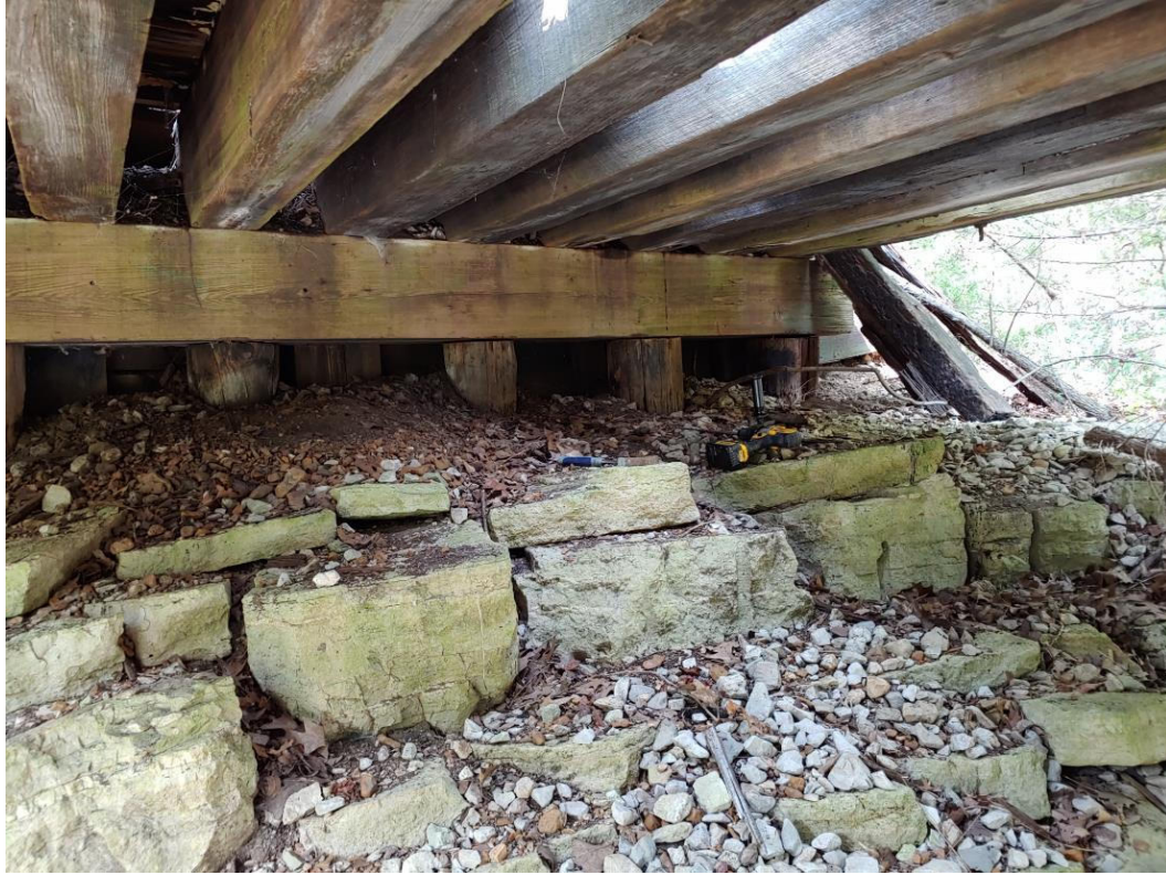
Photo 18 – Existing West Abutment Elevation
