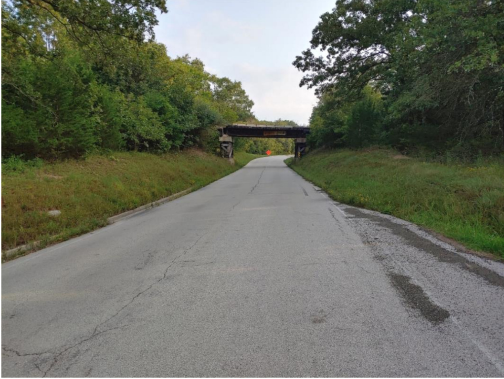
Photo 1 – Bridge Elevation (Looking North)
