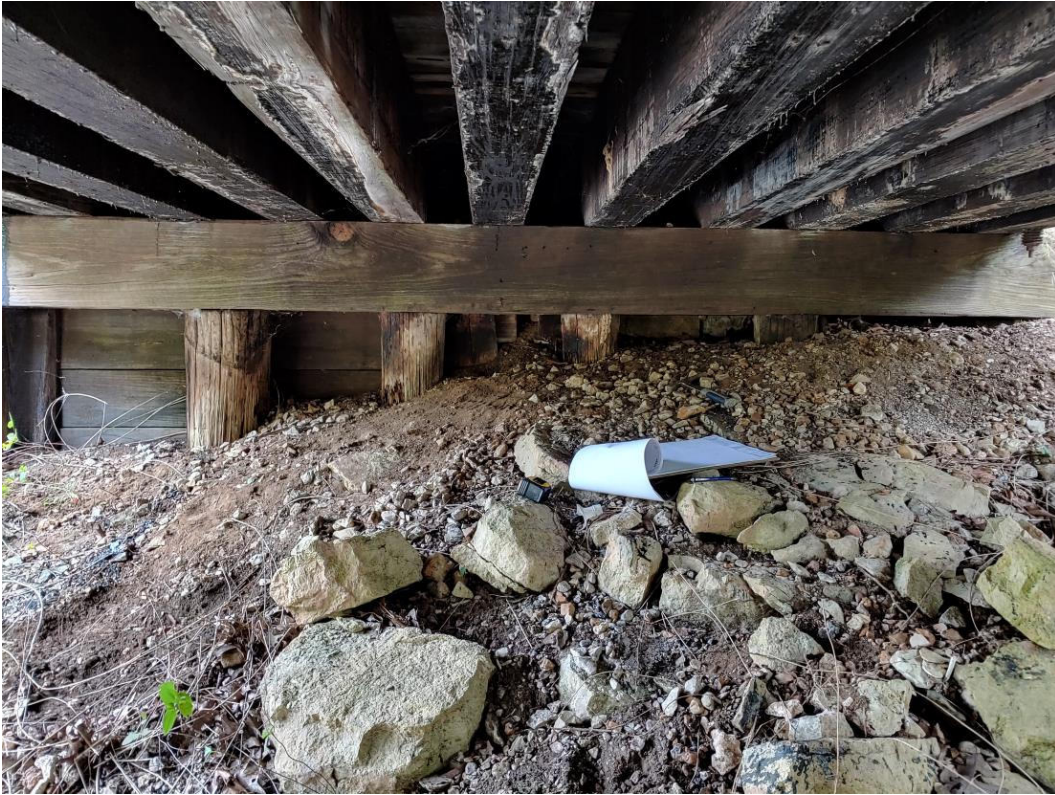
Photo 17 – Existing East Abutment Elevation
