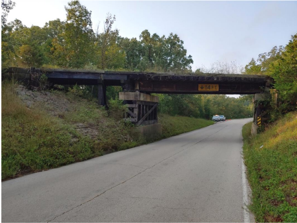
Photo 3 – Bridge Elevation (Looking South)
