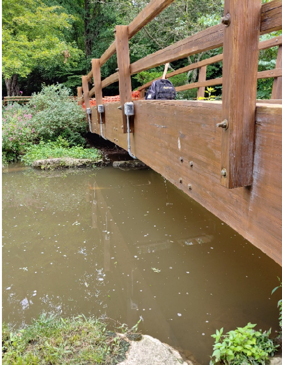
Photo 17 - Typical Railing and Exterior of Glulam
