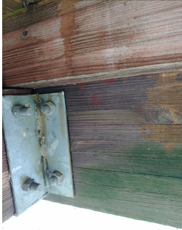
Photo 10 - Typical Floor Beam to Main Arched Glulam Beam Galvanized Steel Connections
