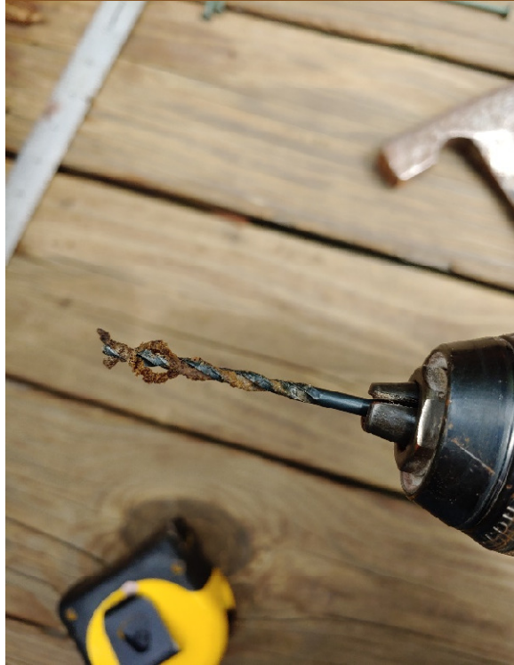
Photo 7 - Main Glulam Soft 1 1/2" when drilled
