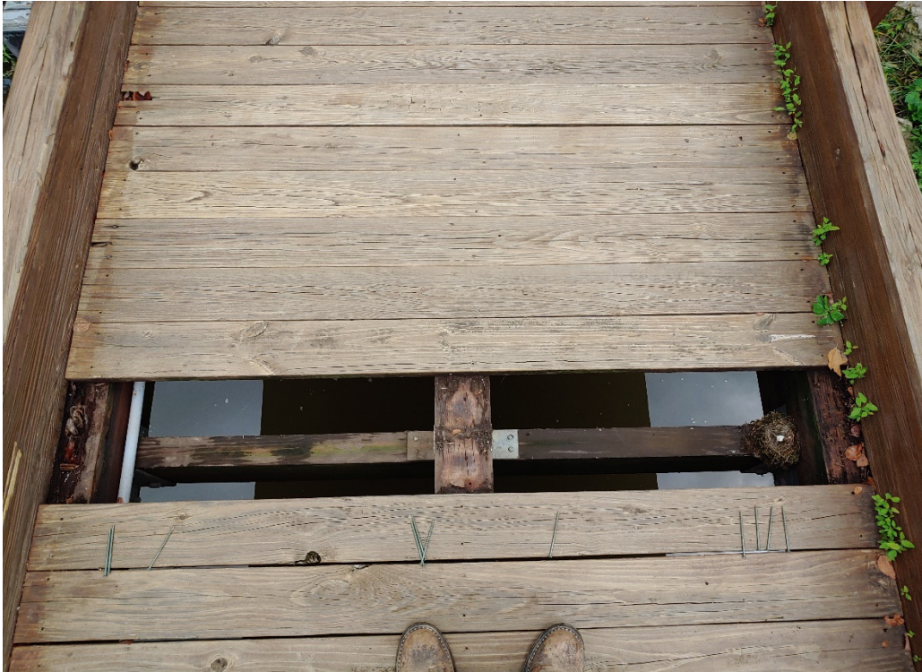
Photo 3 - Typical Underneath of Deck Planks
