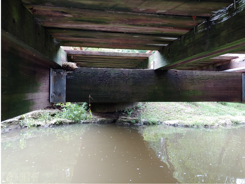
Photo 11 - Typical Underside of Bridge
