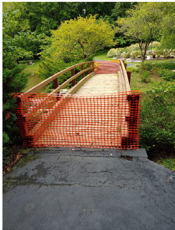
Photo 2 - Top of Bridge Looking West
