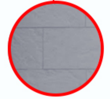
EXISTING EXTERIOR CLADDING
