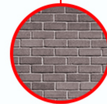
EXISTING EXTERIOR BRICK WALL
